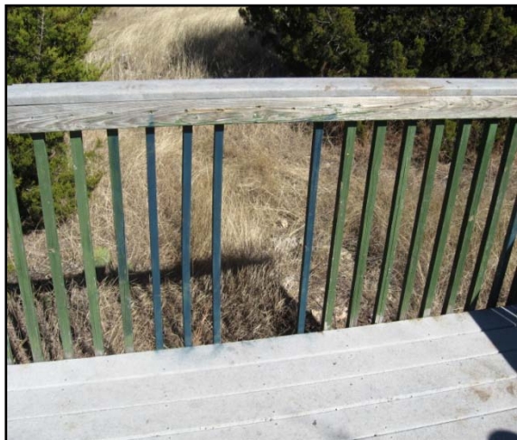
Existing Bat Observation Deck Railing:
