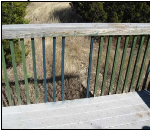
Existing Bat Observation Deck Railing:
