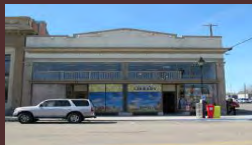
Dewey Building facade built by former Mayor E.H. Dewey
