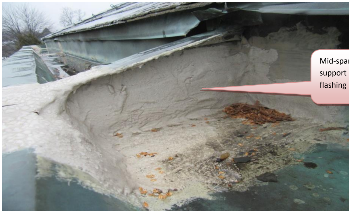
Concealed gutter mid-span support and flashing.
