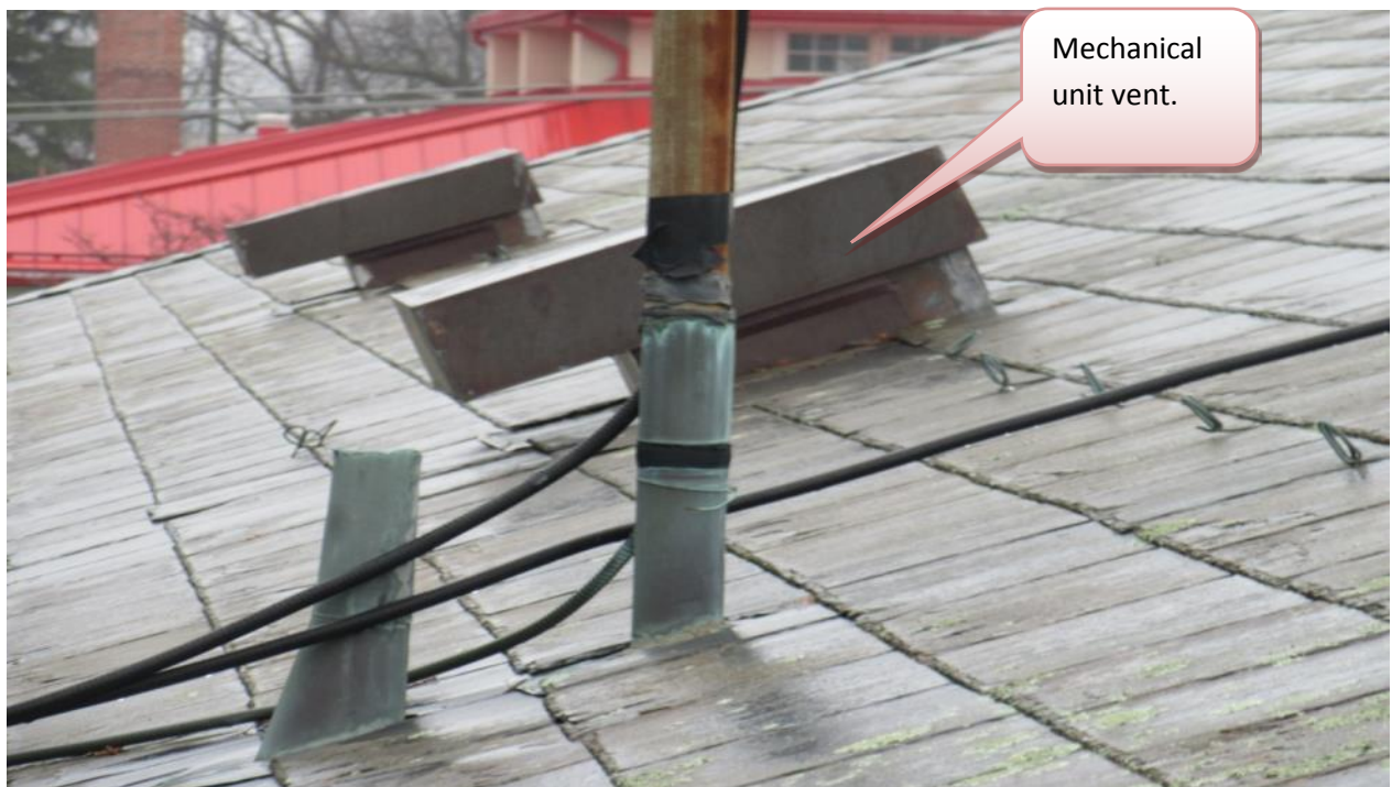
Photograph 10: mechanical unit box vents with crickets. Plumbing vents.
