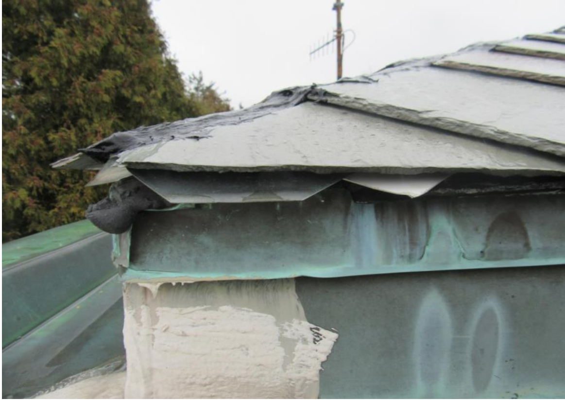
Concealed gutter corner connection and hip roof.
