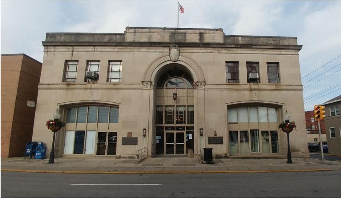
Figure 1: Spruce Street Facade and Parapet on City Hall. 389 Spruce Street Morgantown, WV 26505
