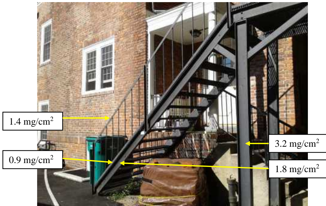
Figure 3 - Community Bldg. Fire Escape
