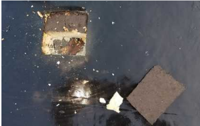
Figure 1- Community Bldg. Roof, Field
