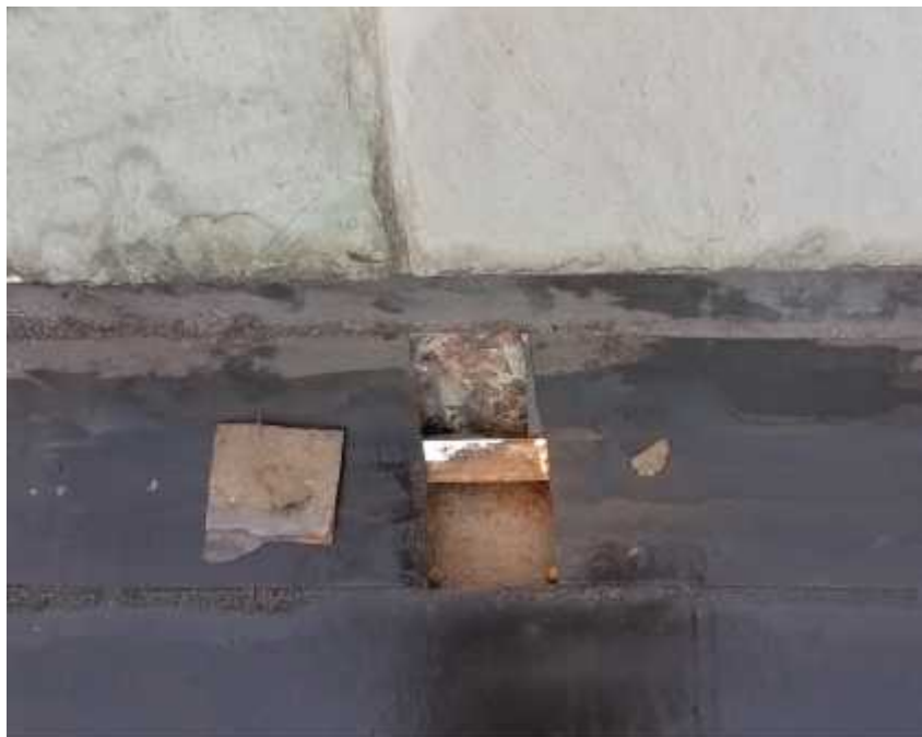
Figure 2- Community Bldg. Roof, Flashing
