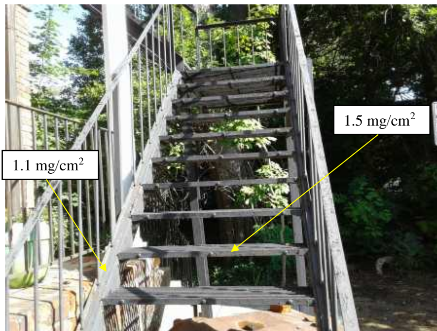
Figure 4- Community Bldg. Fire Escape
