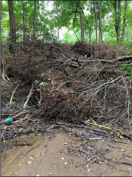
Morningside Drive – Upstream Facing Culvert
