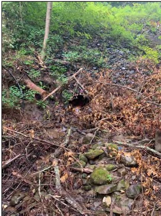
Morningside Drive – Downstream Facing Culvert
