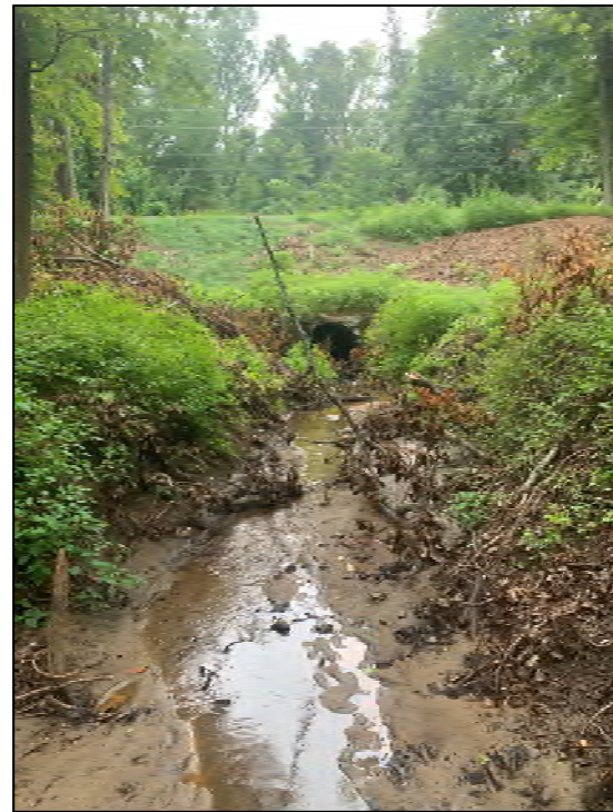
Morningside Drive – Downstream Facing Away from Culvert
