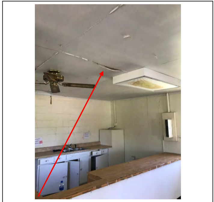
Kitchen 4ft x 8 ft plywood ceiling.
