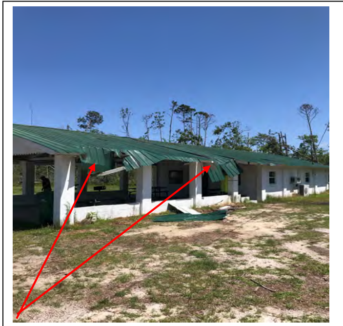
Front View damaged metal roof.
