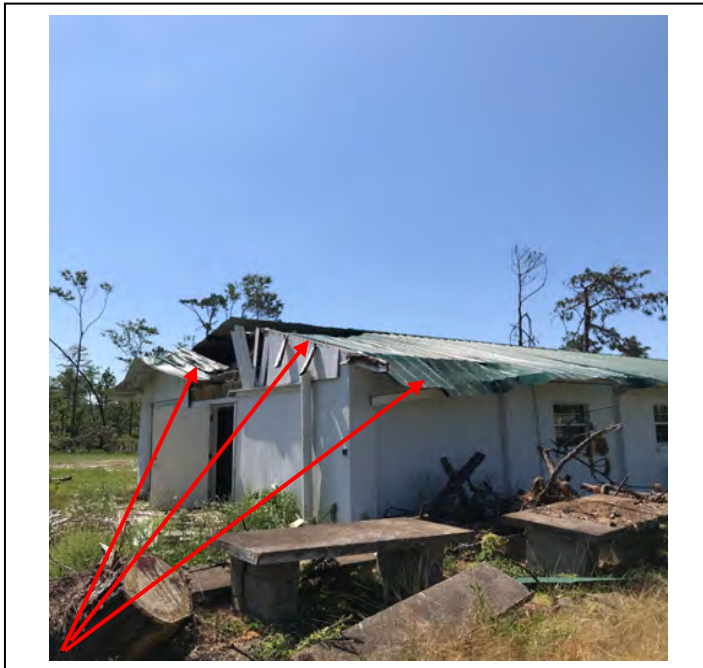
Rear of Building Damage
