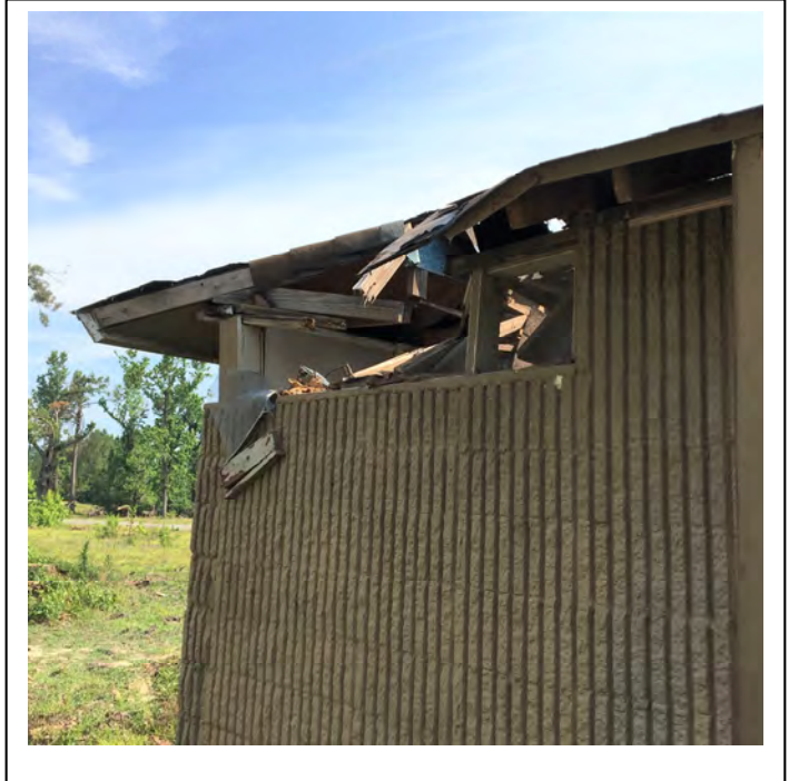
Photo 12: Crushed eave and roof at south west corner.
