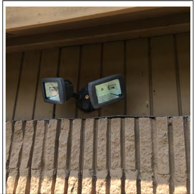
Photo 14: Damaged exterior security light.
