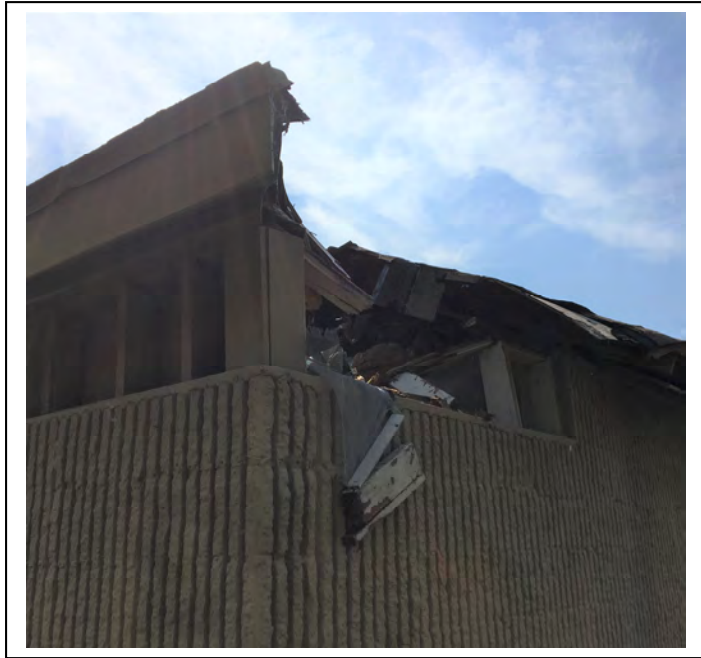
Photo 13: View of crushed eave and screen vent.
