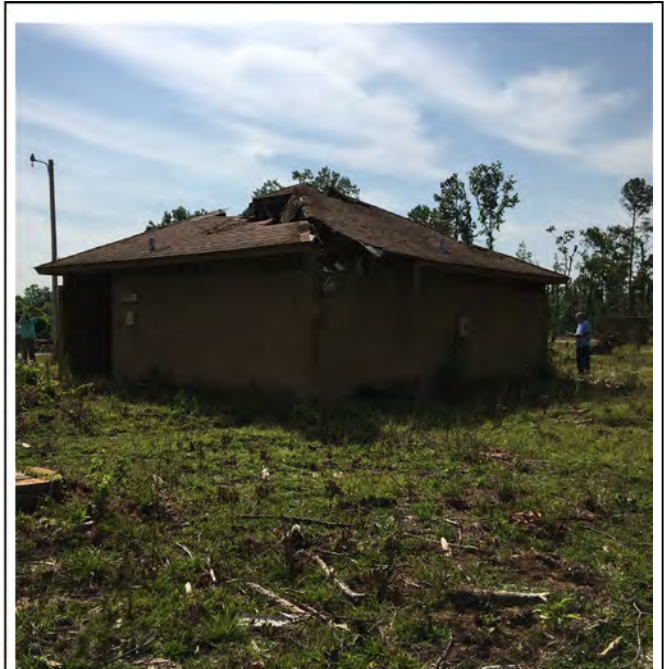
Photo 2: View of west side and south side of building.
