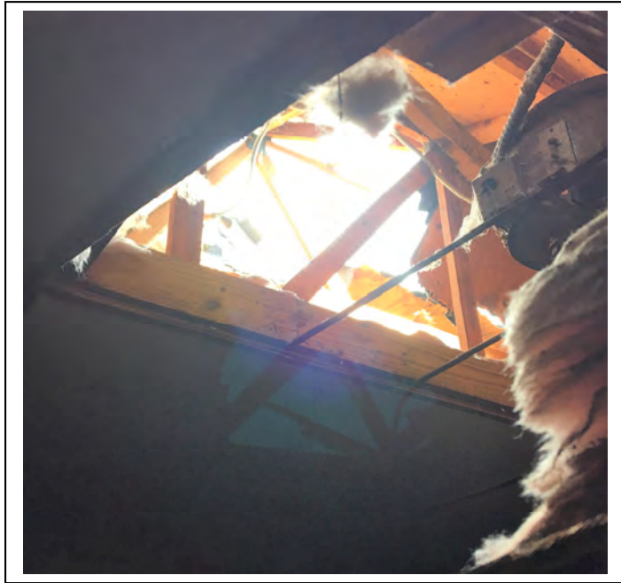
Photo 5: View into attic. Missing and damaged insulation and bathroom exhaust fan
