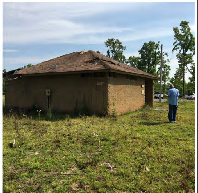
Photo 4: View of south and east sides of building.
