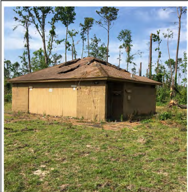
Photo 1: View of north side damage to roof by fallen trees.
