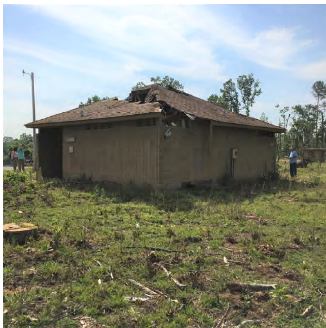
Photo 3: View of west and south sides of building.
