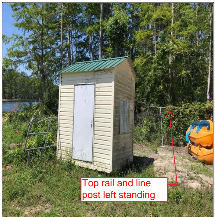
DI 248666 Start 30.79135 -85.140311, End 30.79035 -85.14115, Shows destroyed fence with a few post left.
