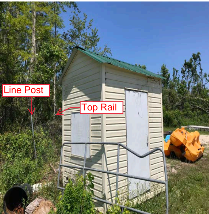
DI 248666 Start 30.79135 -85.140311, End 30.79035 -85.14115, Shows destroyed fence with a few post left.
