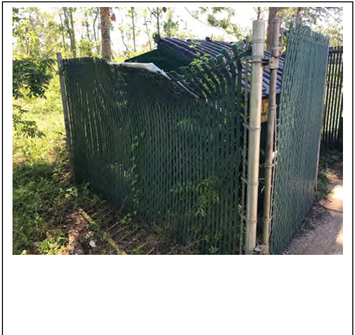
Top rail of chain link fence 2IN (Dia.) X 10FT (L) West side of enclosure bent.
