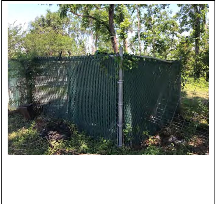
East side of enclosure. Total of 50 slats bent.
