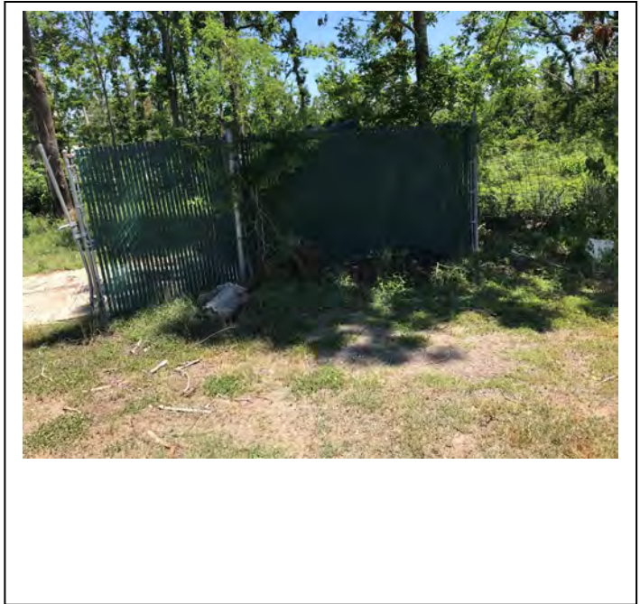
30.79145 -85.14010. Dumpster enclosure gate support pole 2IN (Dia.) X 6FT (L) bent. South side.
