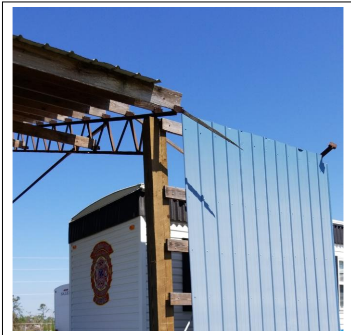
Existing 10 FT wall
