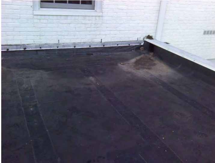
Entry Roof Moisture Noted In Tapered Cricket
