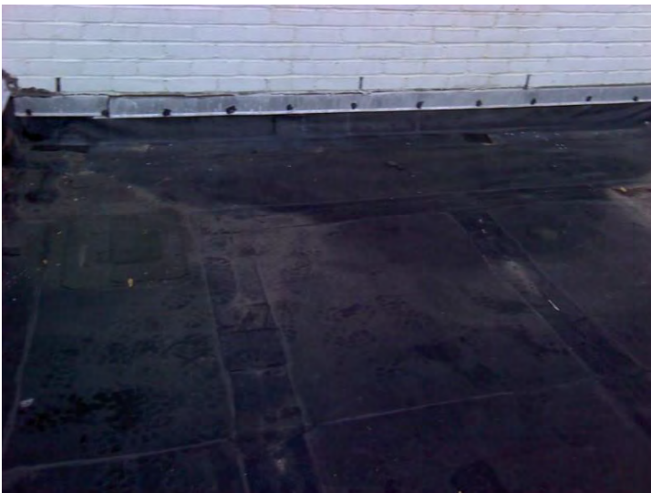
Entry Roof Control Photo Moisture at Wall
