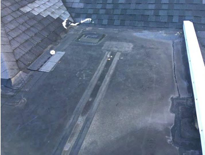
Rear Entry High Point Test Cut By Others - Shingle Tie In - Shingle Debris on Roof
