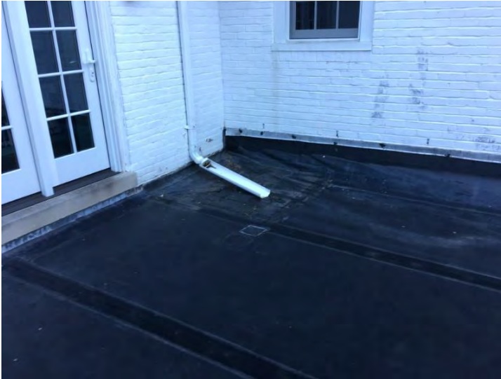
3'-4' From Corner - Moisture Noted During infra red scan (test cut was Dry Insulation)
