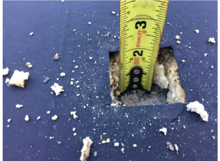
Entry Roof Test Cut - Single Layer EPDM
