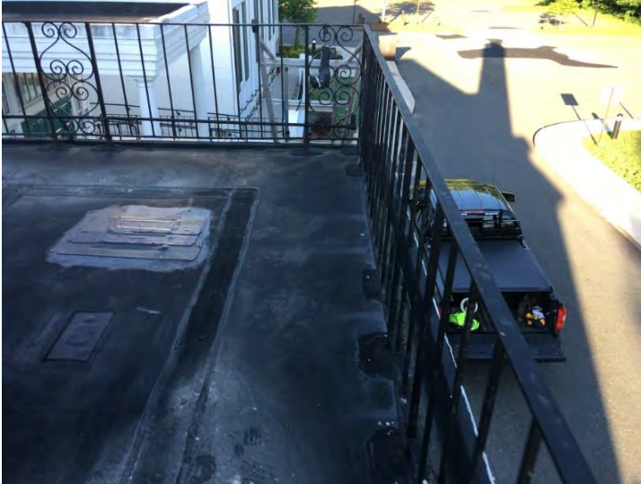
Patio Low Point Test Cut - By Others
