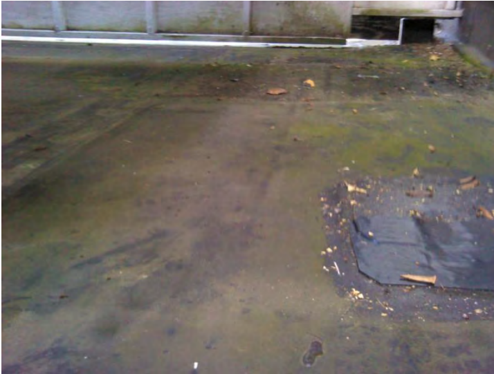
Mechanical Room IR Image Moisture Beneath Membrane Noted on Roof Plan Verified w Test Cut
