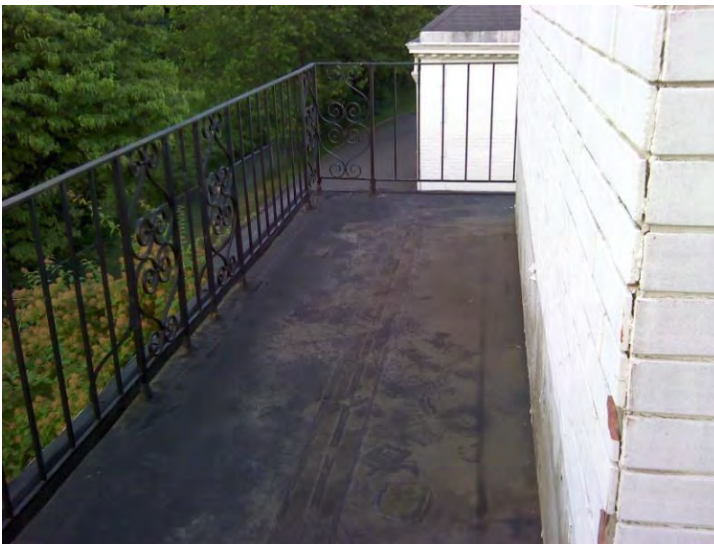
Mechanical Roof Moisture Noted in Corner
