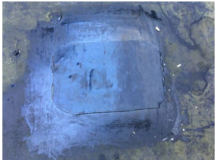
Supreme Test Cut Patch
