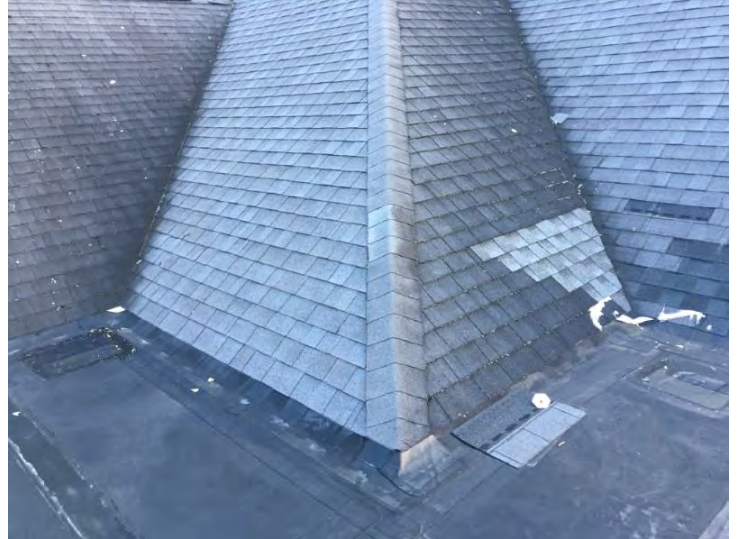
Rear Entry Roof - Shingle / EPDM Tie In
