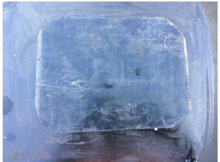
Entry Roof Test Cut Patch
