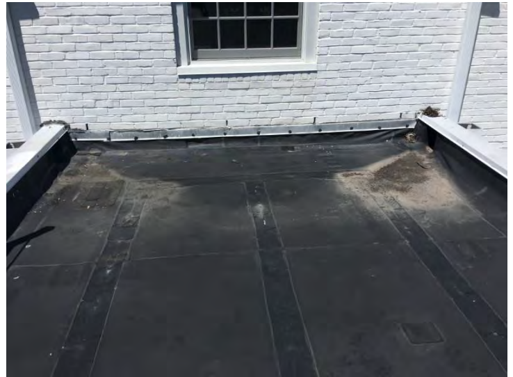
Entry Roof Counterflashing & Cricket Overall (Small Amount of Moisture 2'x2' at Cricket)
