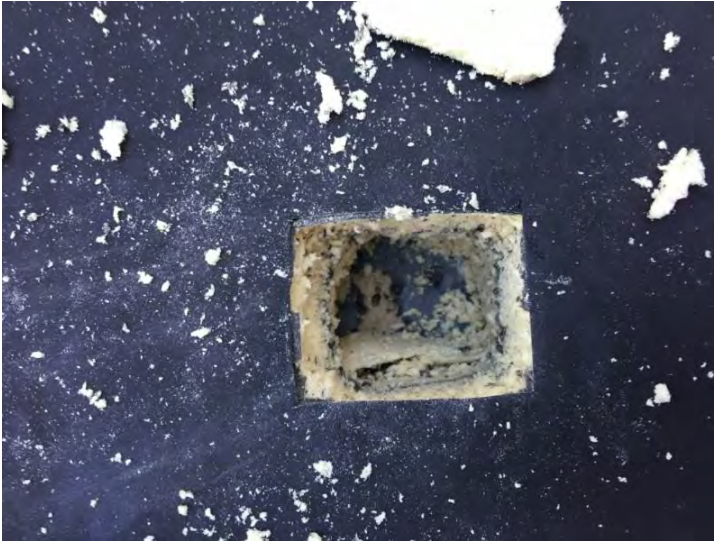
(2) Layers 3.5" Total - ADHERED Insulation & Membrane on Plywood Deck
