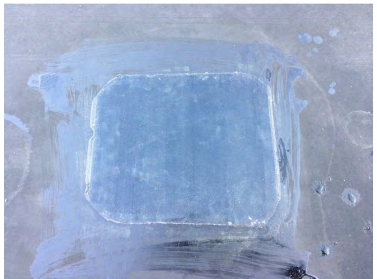
Supreme Test Cut Patch Patio Roof
