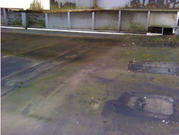
Mechanical Roof Moisture Under Membrane
