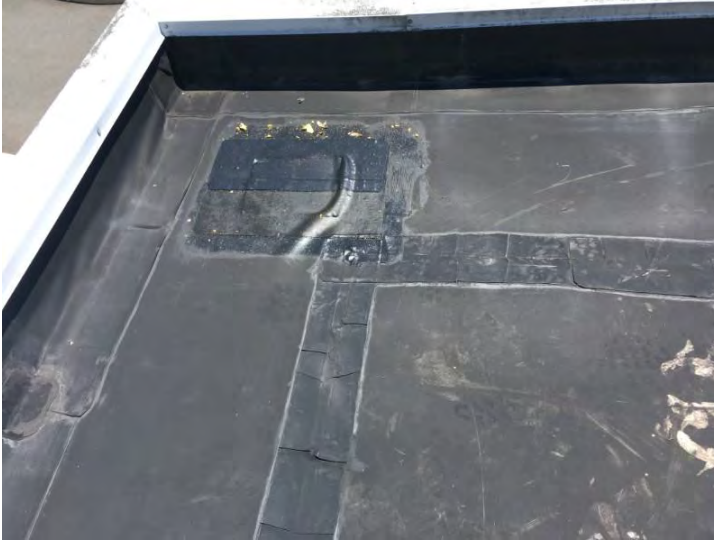
Entry Roof (High Point) Test Cut - By Others
