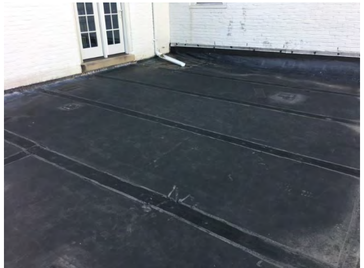
Patio Roof Entry & Corner (DS from Slope Roof) Along Wall & Corner, a small amount of moisture was noted during IR Scan
