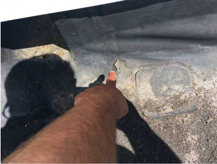
Entry Roof - Failing Patch Near Wet Insulation
