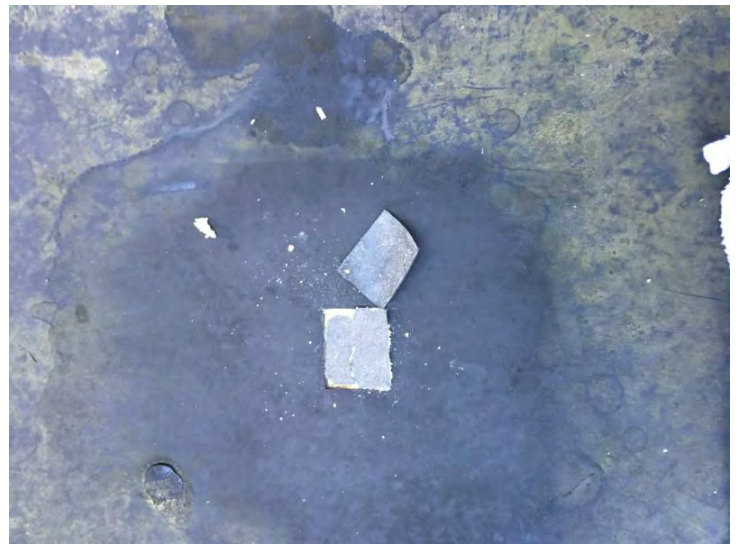
Mechanical Roof - Supreme Test Cut - Surface Moisture under membrane - Insulation = DRY
