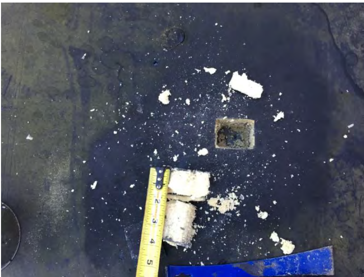
Mechanical Roof Test Cut Composition
