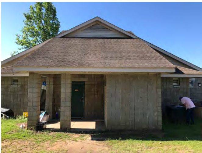
30.79117 -85.14028. Park concession and restroom building. 54Ft (L) X 56FT (W). 6/12 pitch roof. Concrete foundation.
