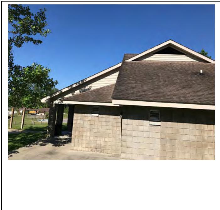
Shingles along the left edge of roof 26FT (L) X 3FT (W). damage to shingles. No apparent damage to under lying roof deck on this one.
