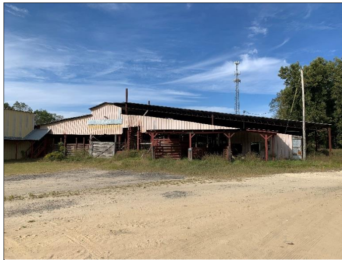
VIEW OF LIVESTOCK BARN
