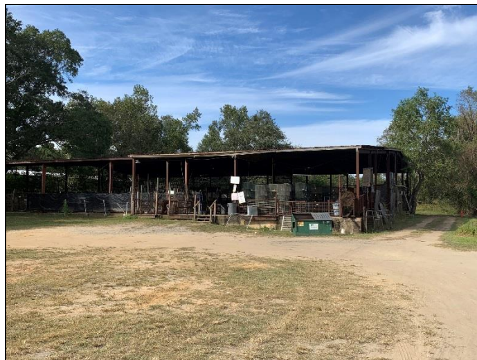
VIEW OF POLE BARN
